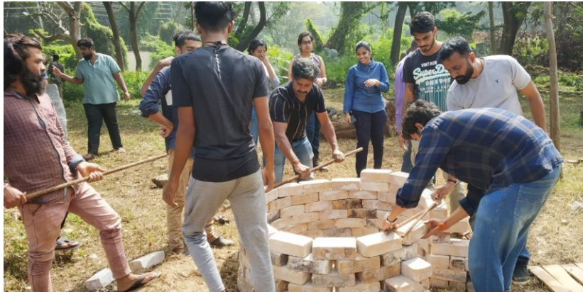
Building a kiln to bake clay artefacts.
